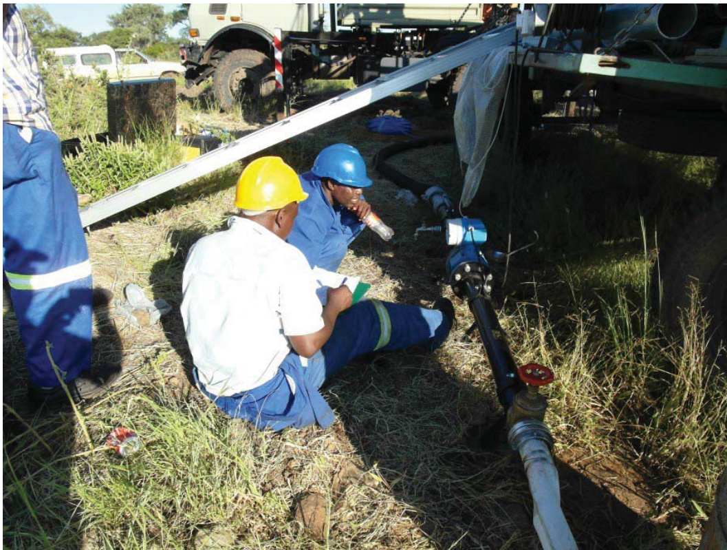
Figure 14: Taking readings from the in-line flow-meter (photo credit: Hans Beekman)
