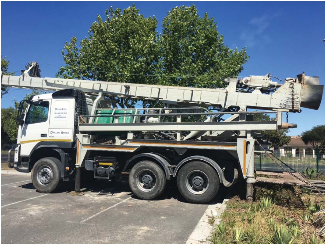
Figure 8: Down-the-hole hammer (DTH) rotary drilling rig
